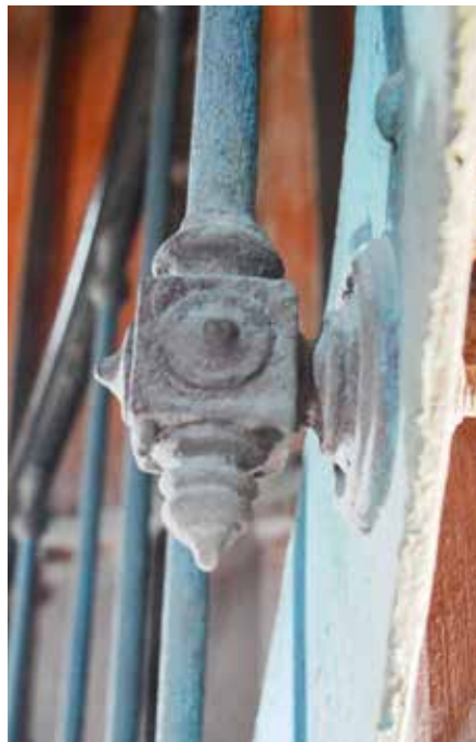
Fastening detail for a decorative element of the stair railing. Photograph: Indrek Laos
