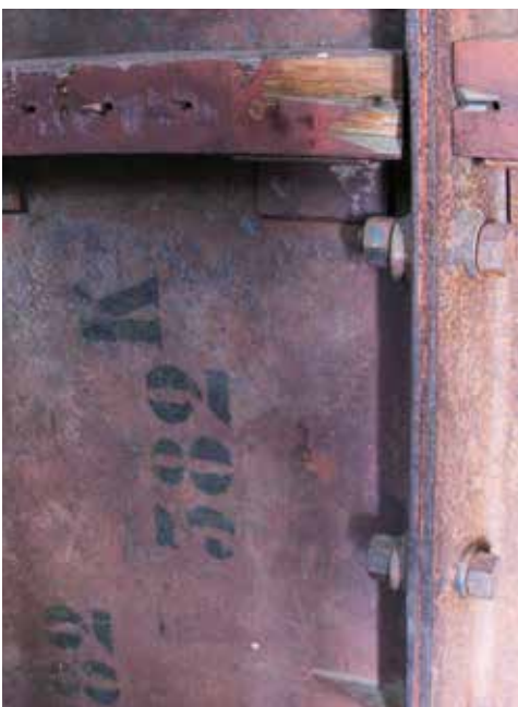
Cast iron plate assembly numbers, July 2015. Photograph: Indrek Laos
